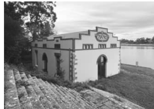
Current state of the theatre, in May 2025.
